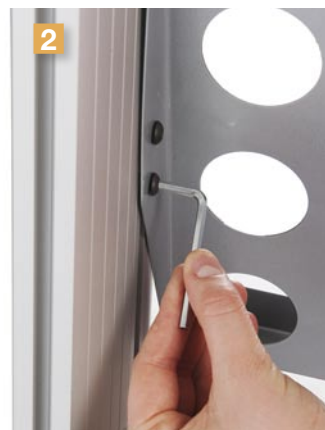
Lock the screws with the allen key
